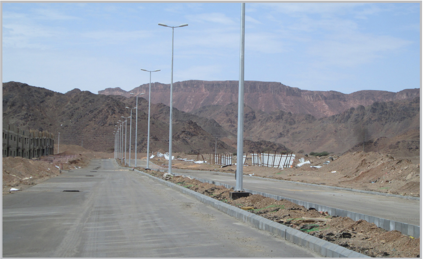
Lighting installation project - Khaybar
