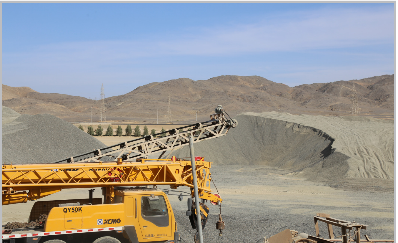
Crusher Project at Al-Ula
