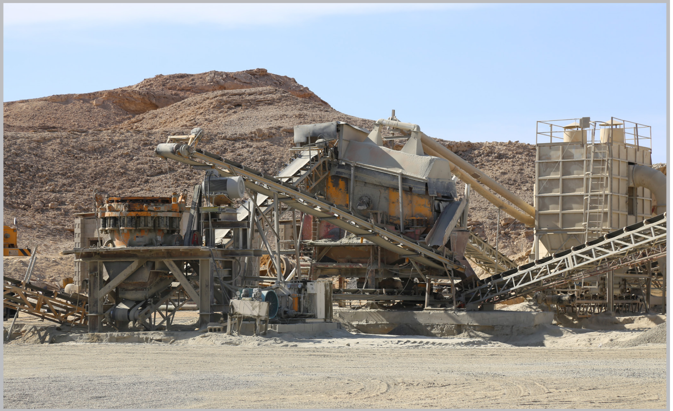
Crusher Project at Al-Ula
