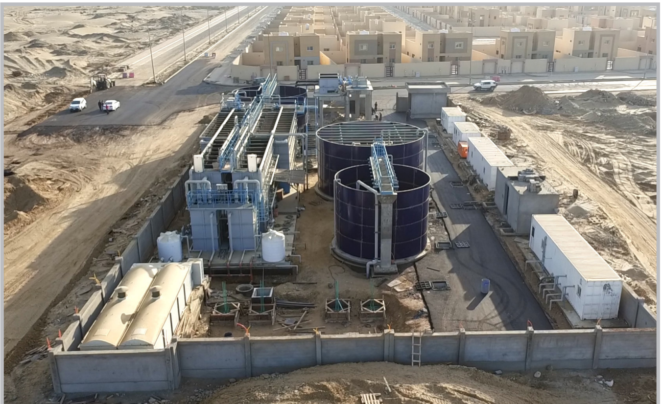
Station Works - Al-Khurma
