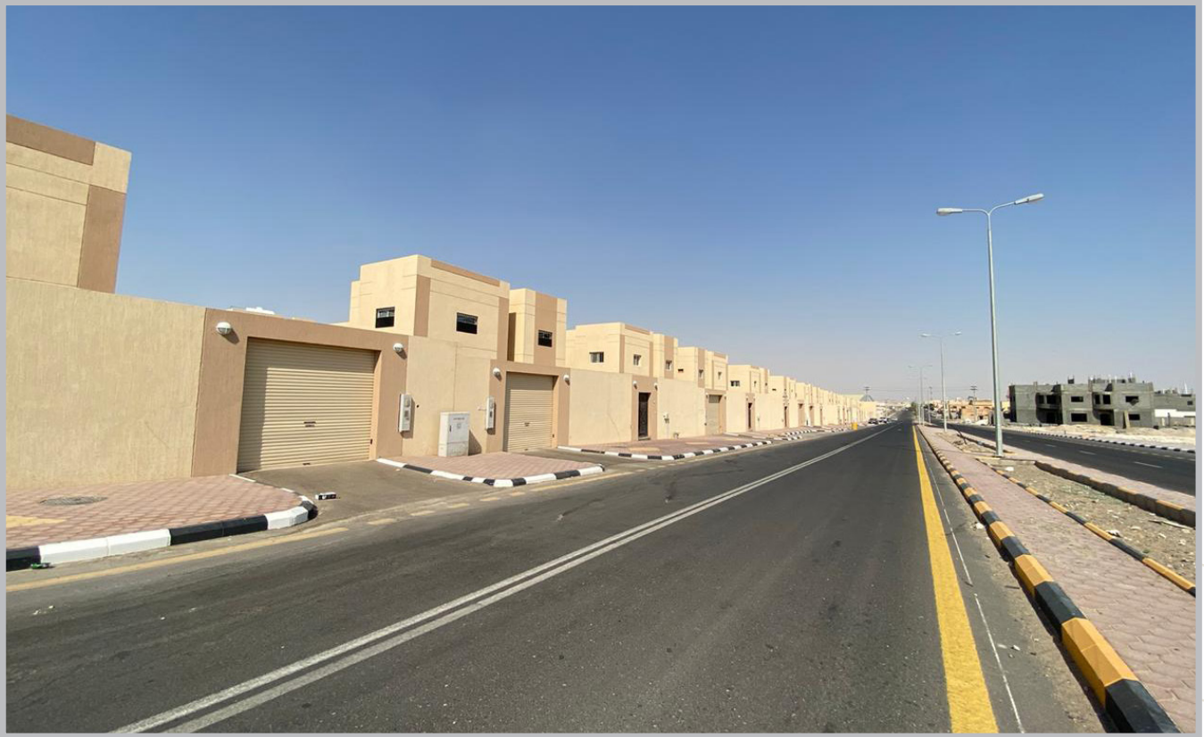
Buildings Maintenance -Tabuk
