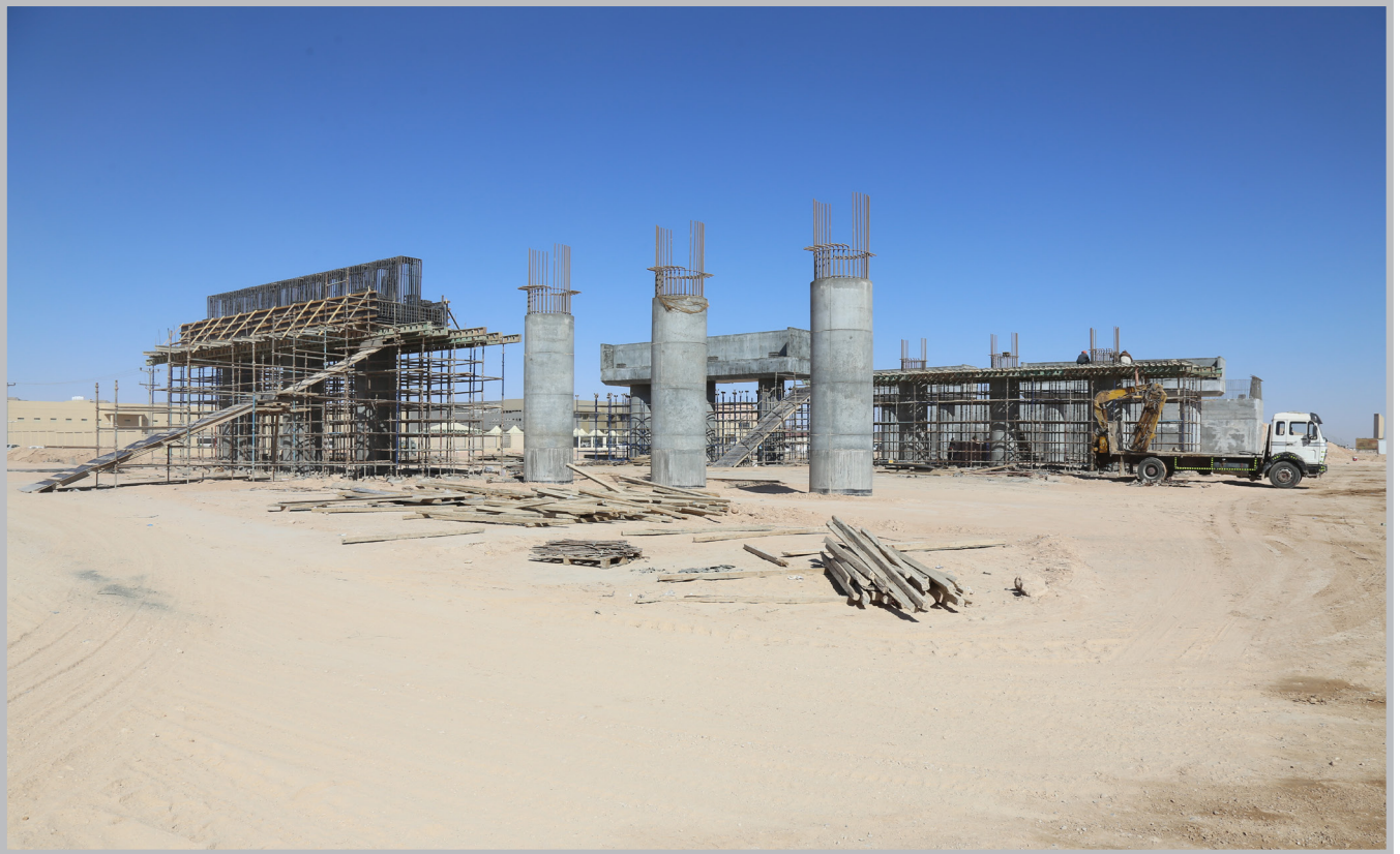
Bridge works - Hafar Al-Batin
