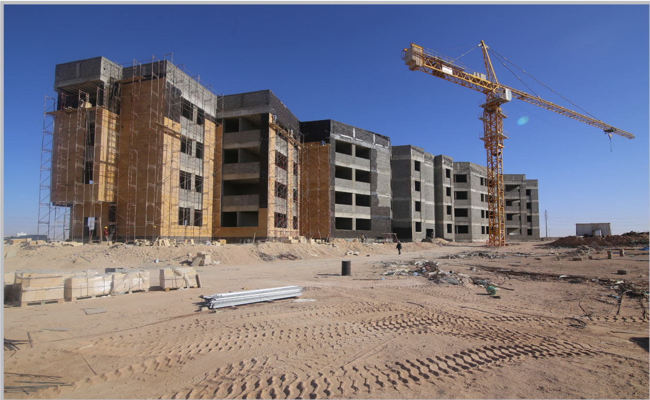
Bridge Works --- Hafar Al-Batin Municipality Building
