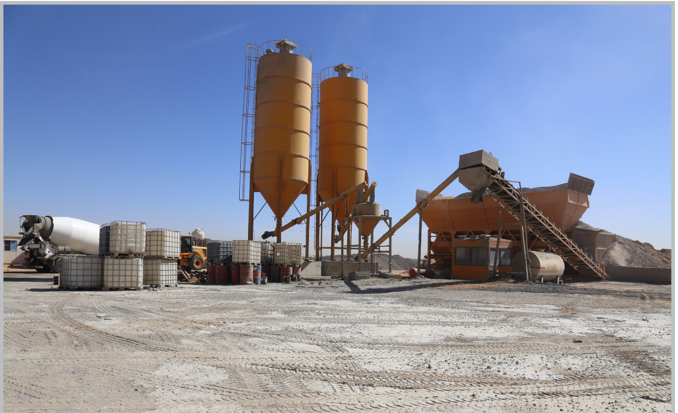
Production Units for Bridge Works - Hafr Al-Batin
