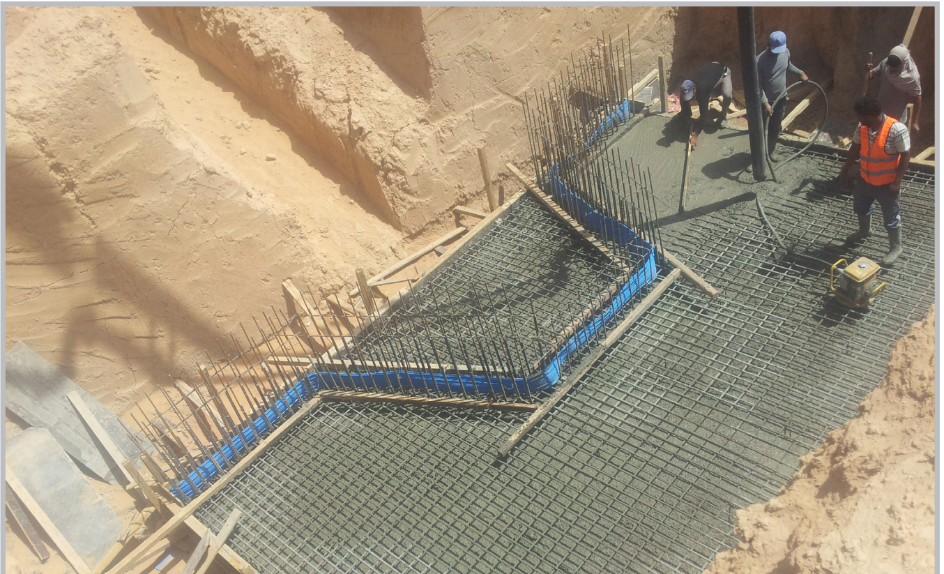
Manhole works - Khaybar
