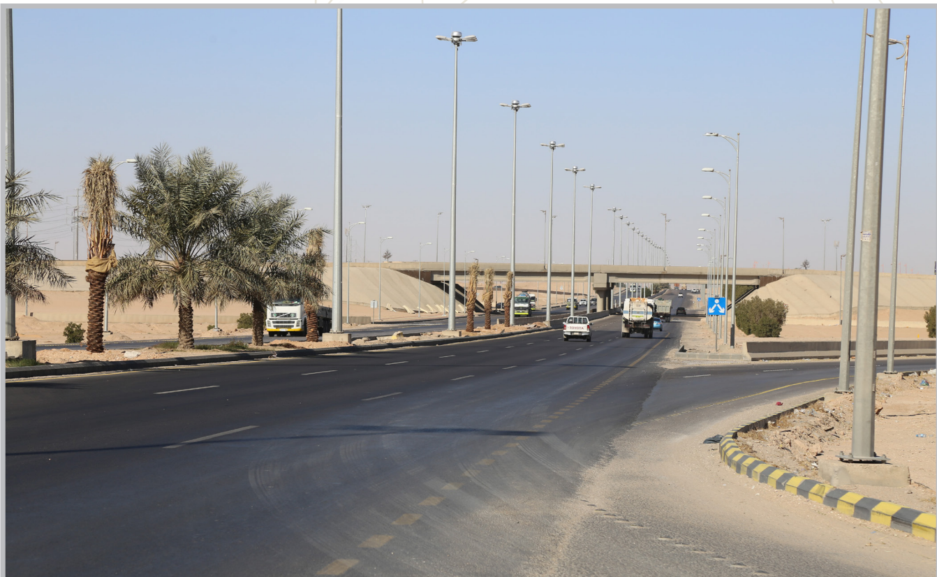
Asphalt works - Hafar Al-Batin
