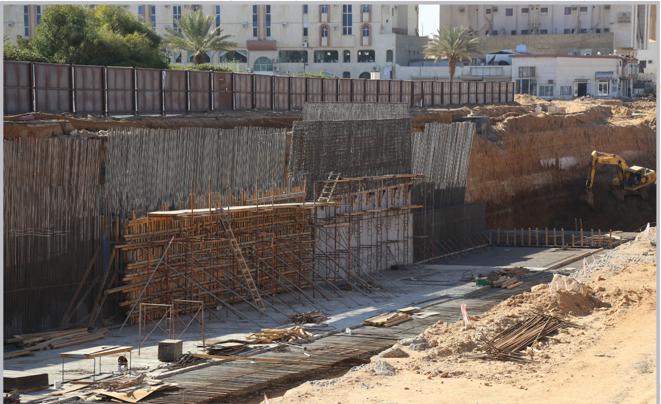
Bridge Works - Hafr Al-Batin
