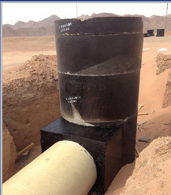
Water Networks - Khaybar
