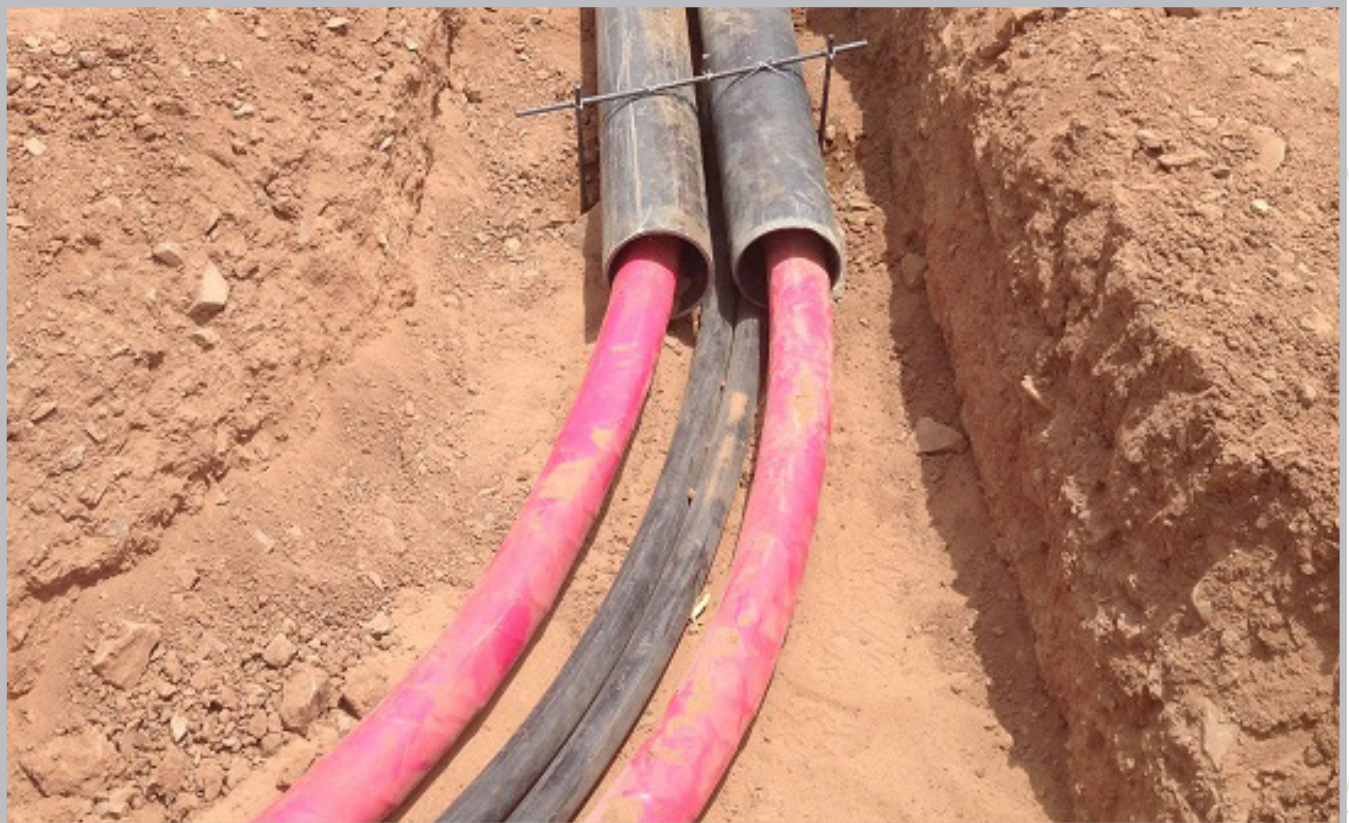
Cable Backfill Works
