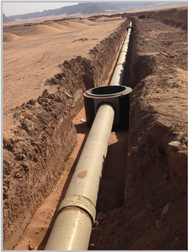
Water Networks - Khaybar
